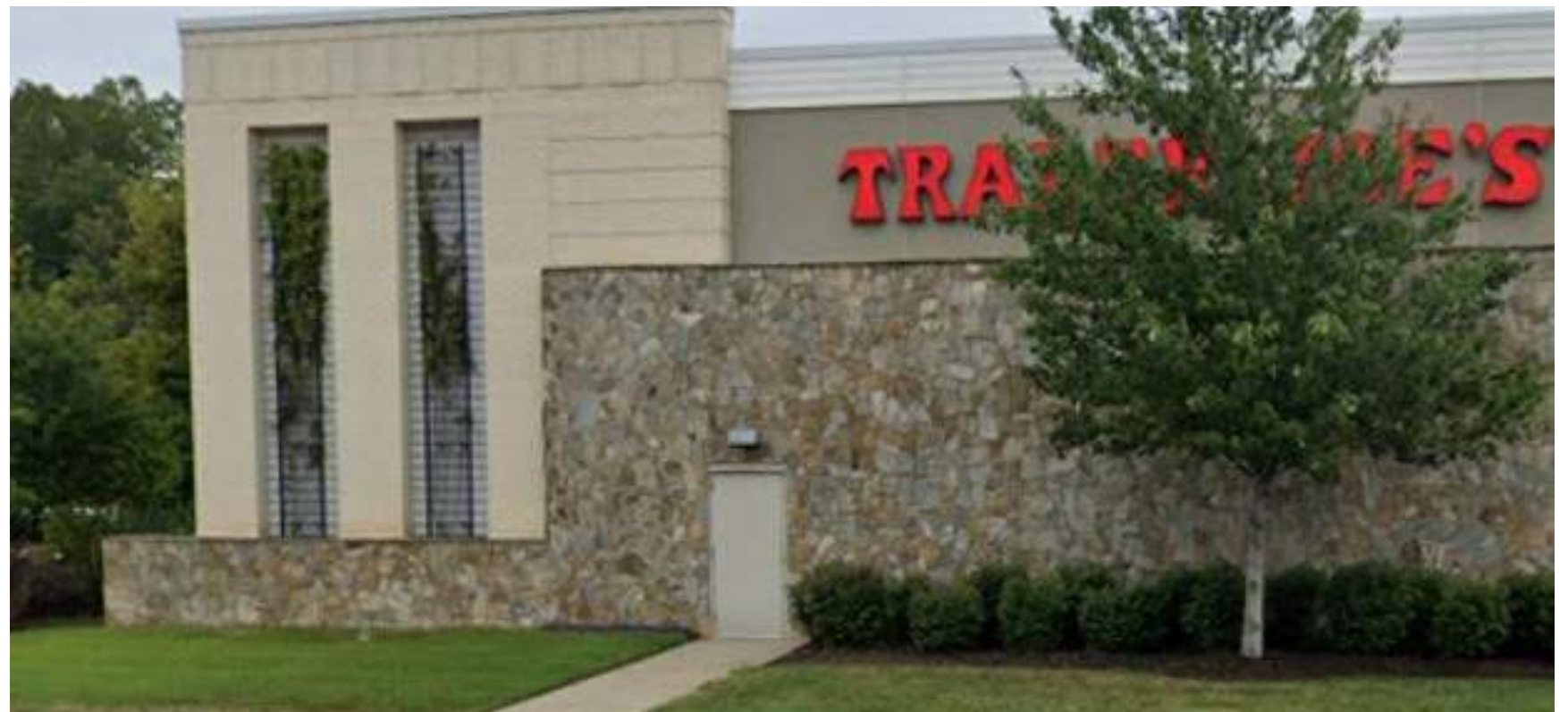
3 | TRADER JOE'S - GREEN SCREEN IN RECESSED PANEL OF SIDING
