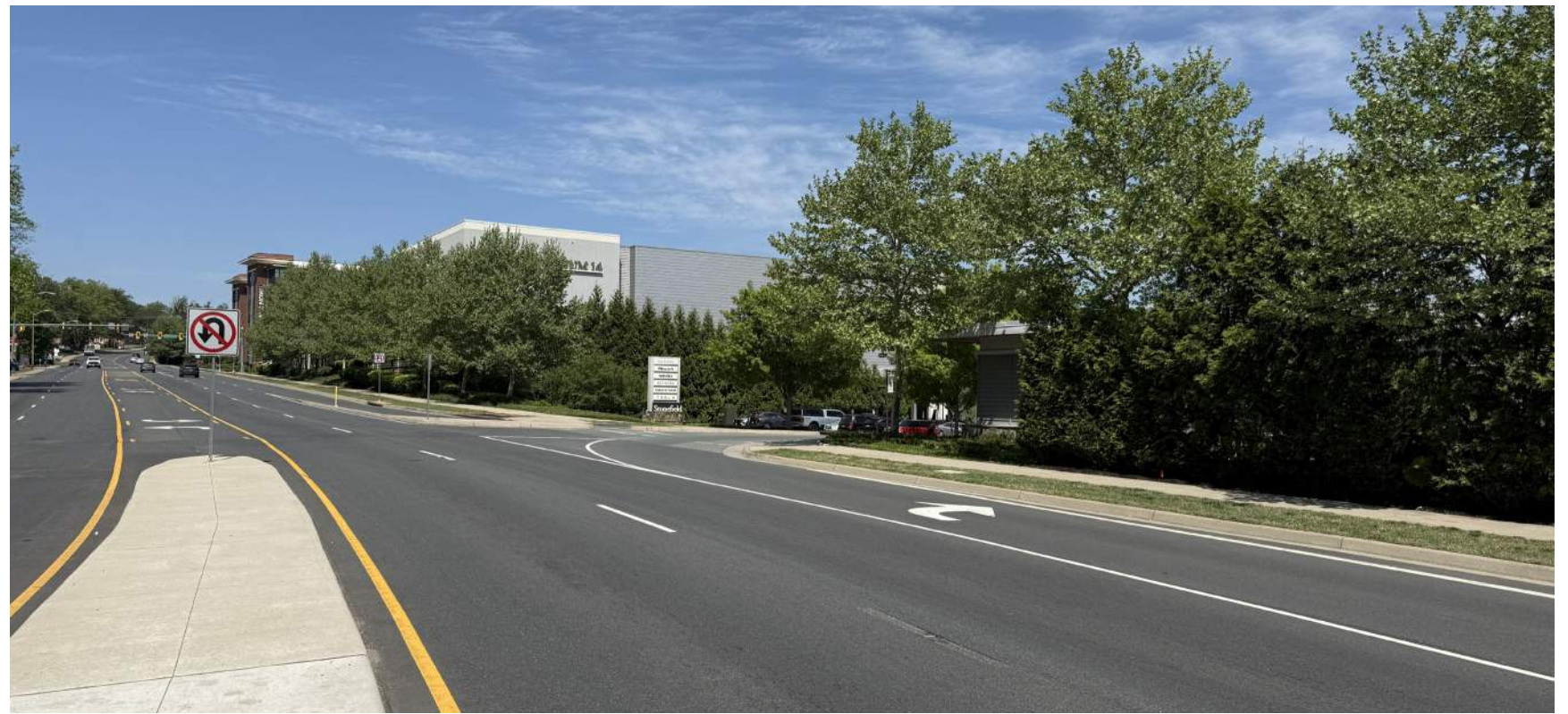
VIEW OF SITE FROM HYDRAULIC RD NORTHBOUND
